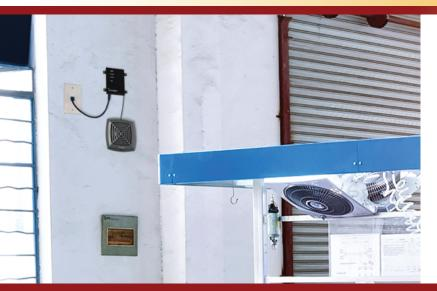
The Network Relay Controller with Horn-Buzzer utilizes a network based time source via PoE or LAN connection, enabling signaling of one or multiple Horn-Buzzers. Activation and synchronization of all timed and coordinated events is performed using pre-programmed scheduling software.
